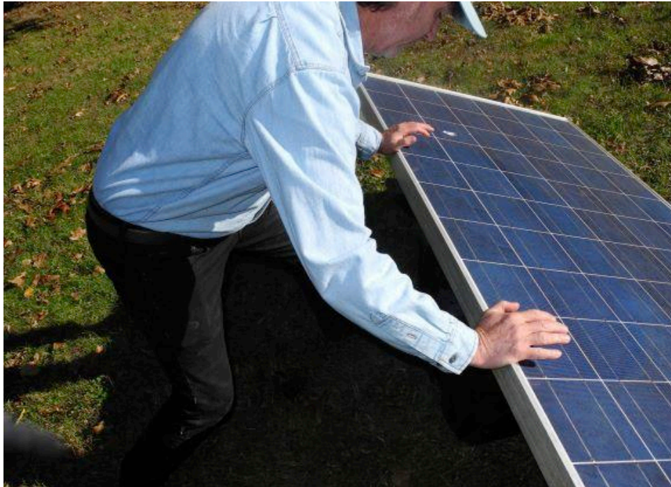
Figure 15. Worker pushing panel down into slots.
