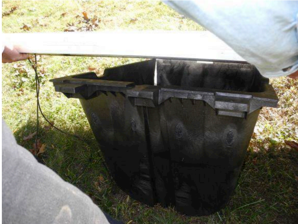
Figure 13. Worker lowering the panel onto the high side tabs
