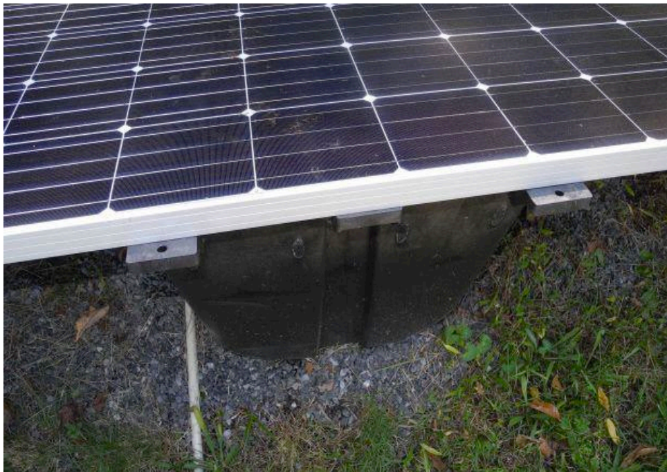
Figure 16. Panel fully seated in the PowerRack high side slots.
