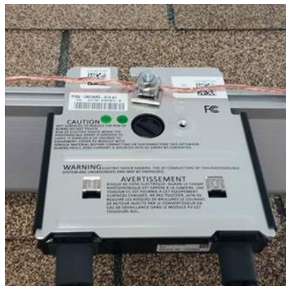
Figure 3: Grounding lug
